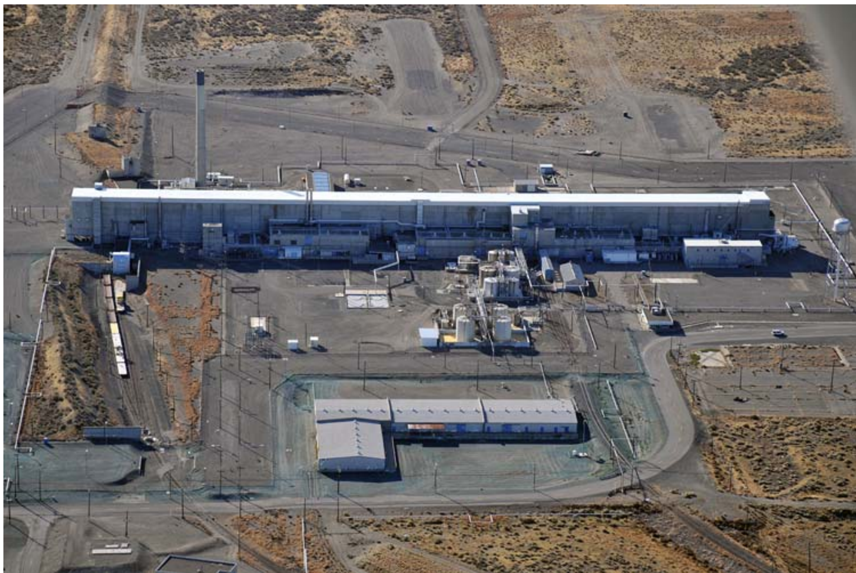
Figure F.6-3. PUREX Plant and Tunnels to South (above the plant in photo)
